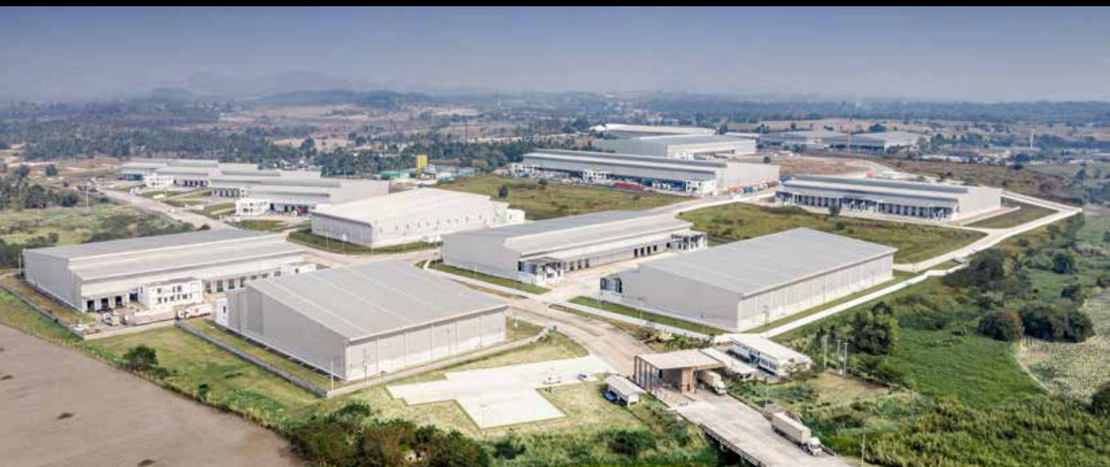
Frasers Property Logistics Park (Sriracha), Chonburi, Thailand
