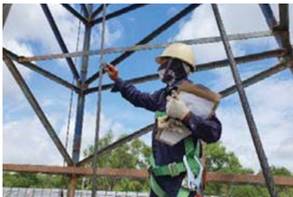
Photo of contractor’s PPE for work in height
