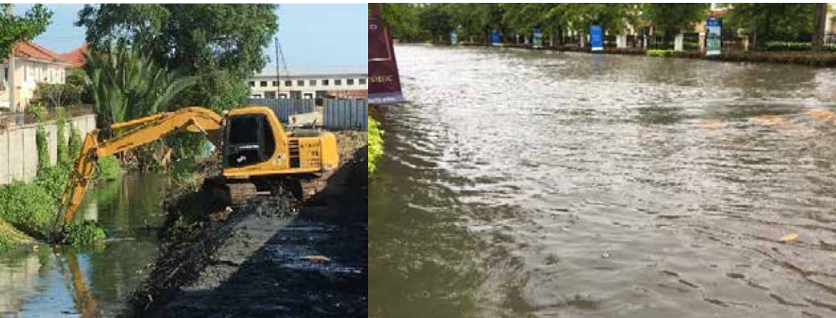
▲ The activity for dredging canals around the Grand Rama 2 project.
